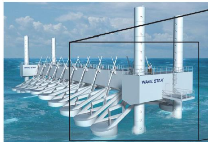
Fig. 3 Commercial converter with 20 floats (left) and test-section at Hanstholm with two floats (right)
